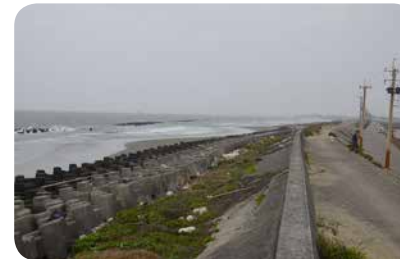
▲圖2-72 浮洲中段堤防前的離岸堤
